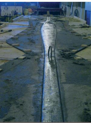
Full-scale fabric formwork beam cast, 2003
